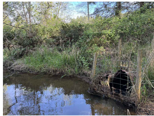
3 OLD WAGON ROAD CULVERT UPSTREAM INLET WITH TRASH RACK Scale: NTS
