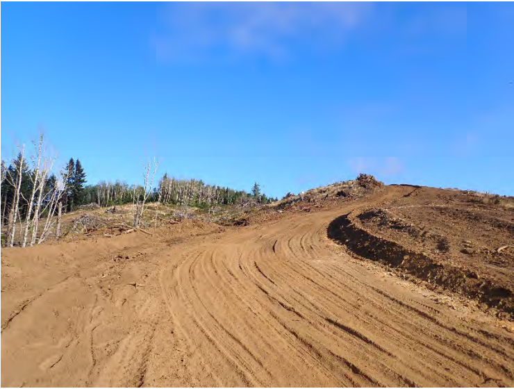
Looking up slope along the proposed gravel drive.
